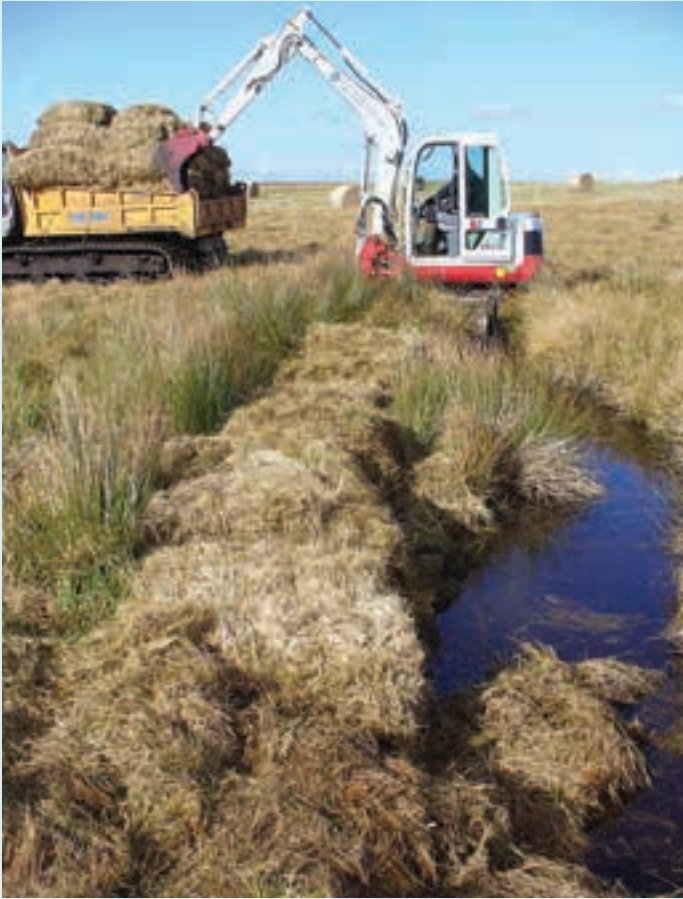
Figure 5.4 Ditch restoration on Exmoor: slowing water down by re-wetting moorland
